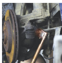
Loosening track rods
