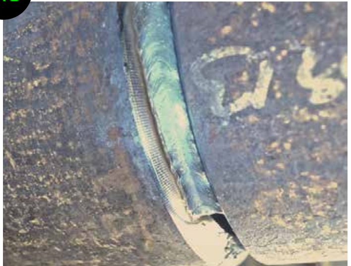
IAC - Vertical downward welding of a root pass in a district heating pipe. Welding speed is significantly increased compared to traditional upward welding..
